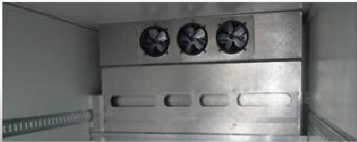
Figure IX-3. Cold Plates and Blowers
